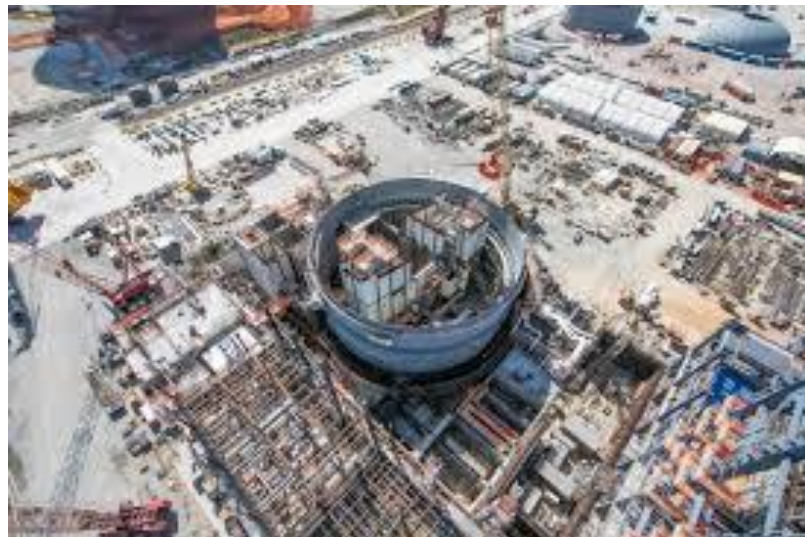
Construction of Calandria wall
